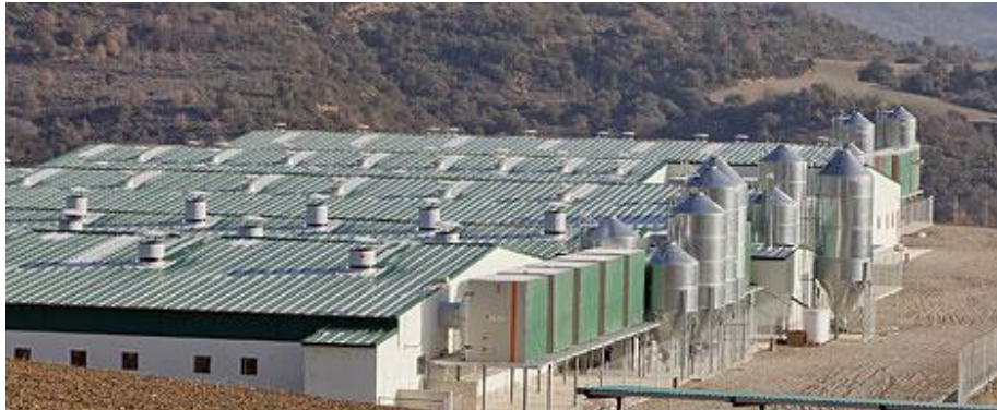
AirProTec filtration units installed in a breeder farm in Spain
